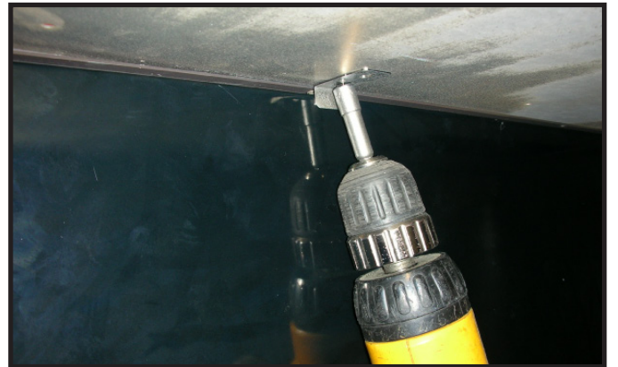
Figure 6. Installing Angle Tab to Secure Inner Back Panel.
